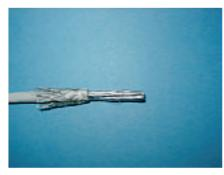
STEP 4: Pull back load-bar toward insulation. Maximum gap: .078" / 2 mm
