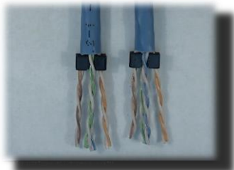
5A. NOTE: Center pair colors change position depending on the cable end being terminated.
