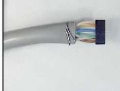
13. Wrap drain wire around cable jacket.
