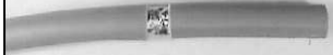
2. Place boot over cable jacket if required. Cut cable jacket approx. 1 1/4 inch.
